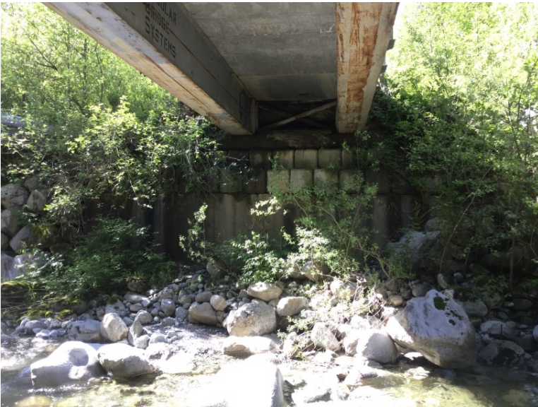
Right Bank Abutment when facing downstream
