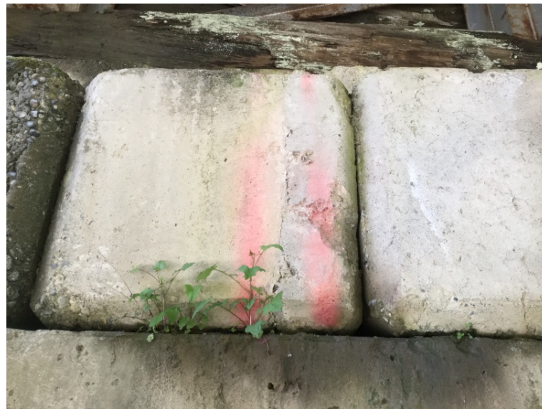
Lock block on right bank abutment
