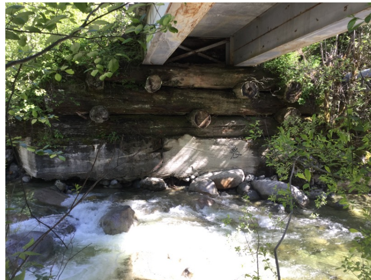
Left Bank Abutment when facing downstream
